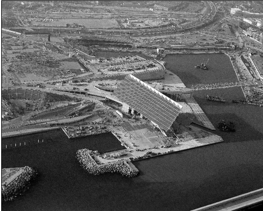
Image 4.- Aerial View of FORUM PV Pergola
