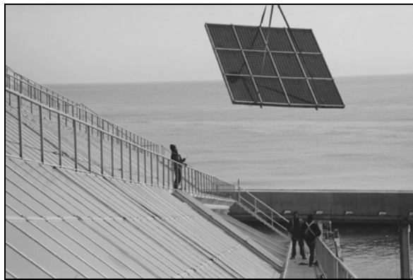
Image 2.- Installation of set of 12 modules
